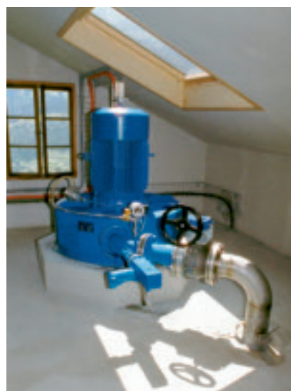
Fig. 5 Turbine Pelton 75 kW.
